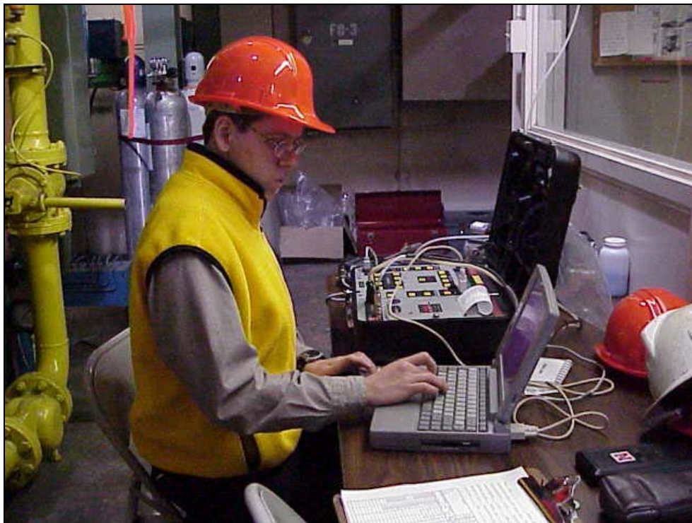
Fig. 14. Logging of emissions data from Enerac 3000E.
