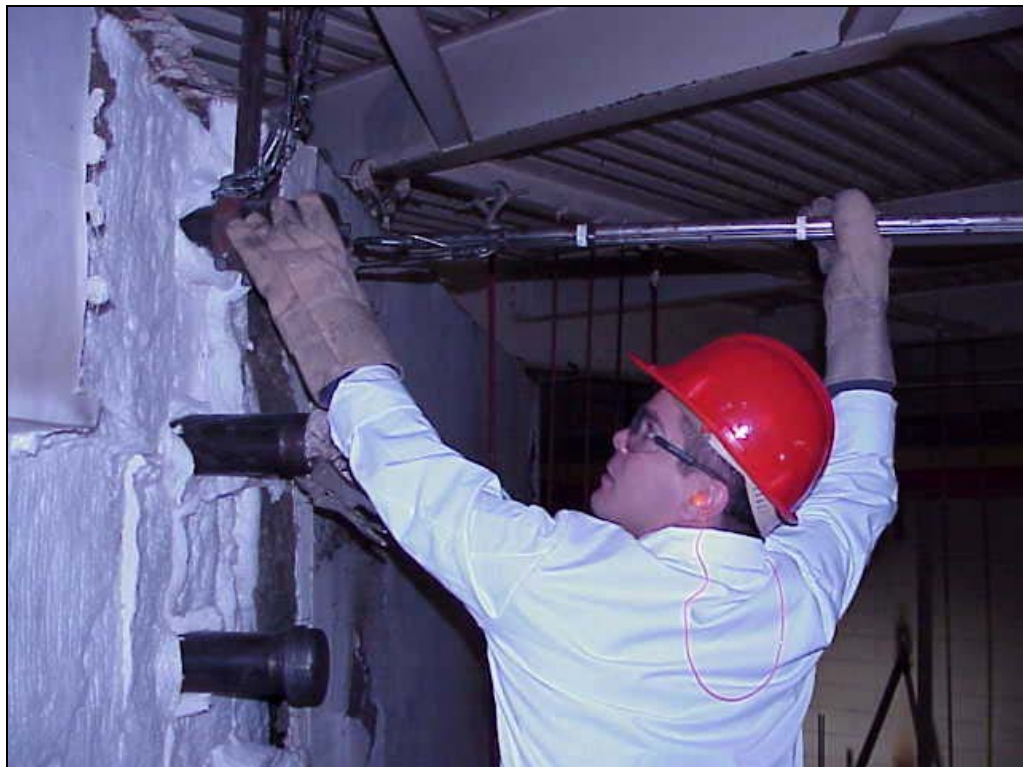
Fig. 12. Inserting particulate testing probe into breaching.
